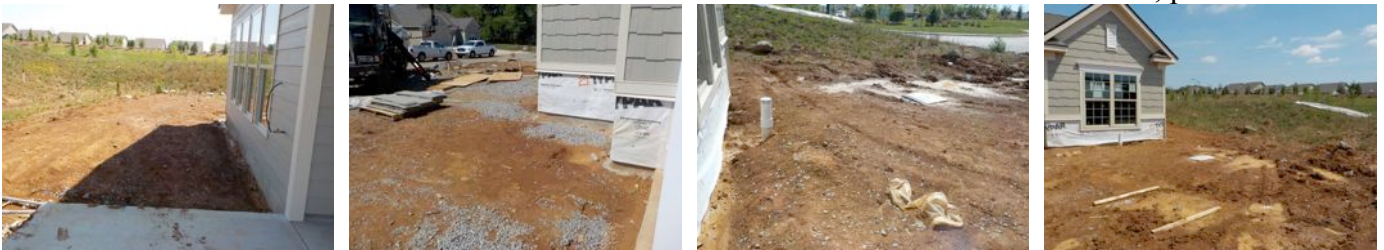
Water Penetration Due to Subgrade Soil Conditions
